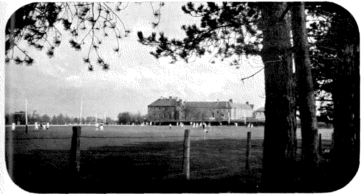
VIEW OF HOUSE FROM GROUNDS
